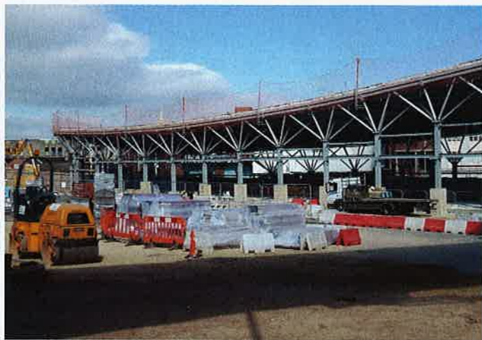
Planning issues resolved, construction got under way in November 2011
