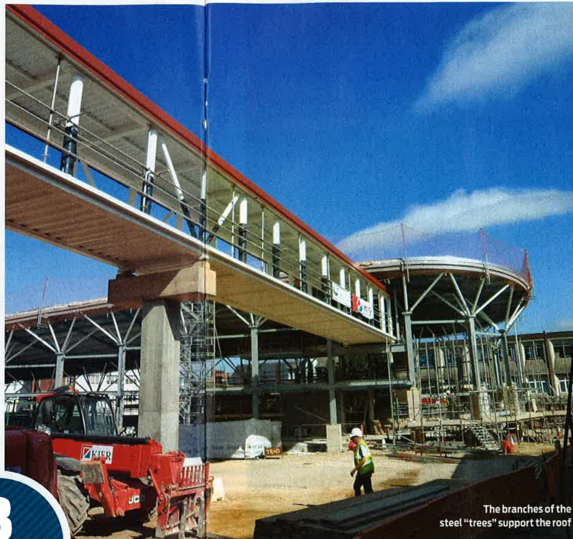
The link bridge was placed on its bearings in two sections
