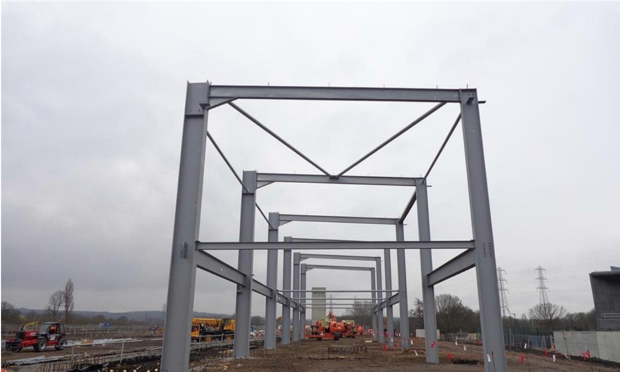
Thameslink Depot - Three Bridges, Crawley
