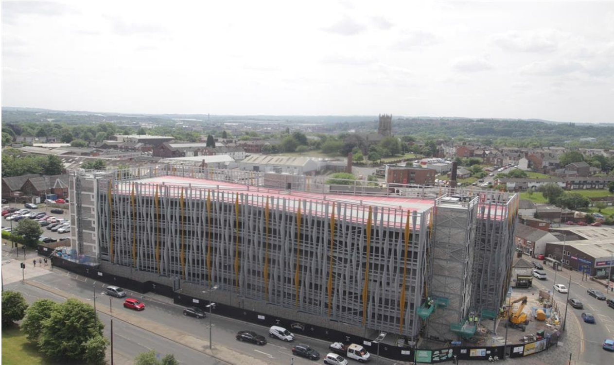
Smithfield Multi-Storey Car Park - Stoke-on-Trent
