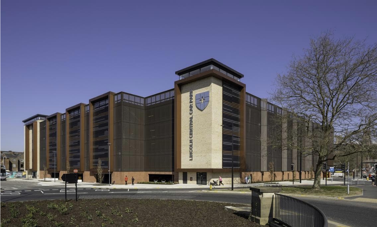
Lincoln Transport Hub - Car Park
