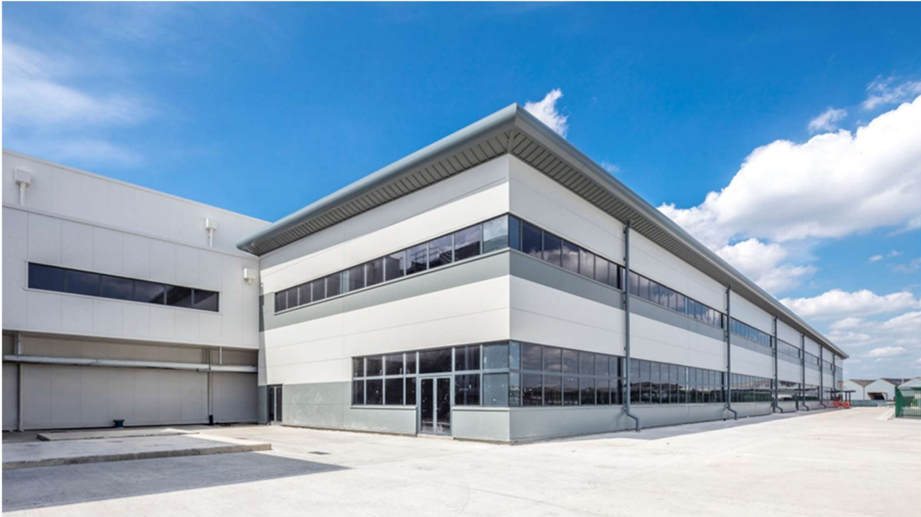
Project Dragonfly, Ocado - Multi Temperature Warehouse, Erith
