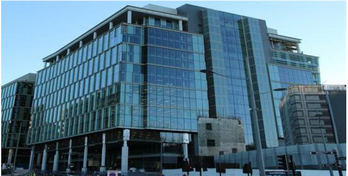
Snow Hill 2 Building, Birmingham City Centre
