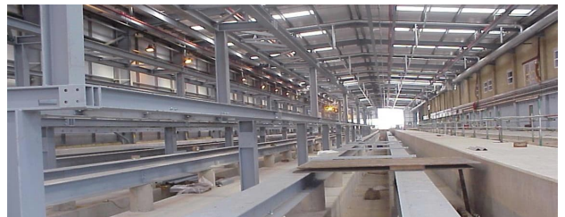
(Siemens Train Care Facility - Southampton)
