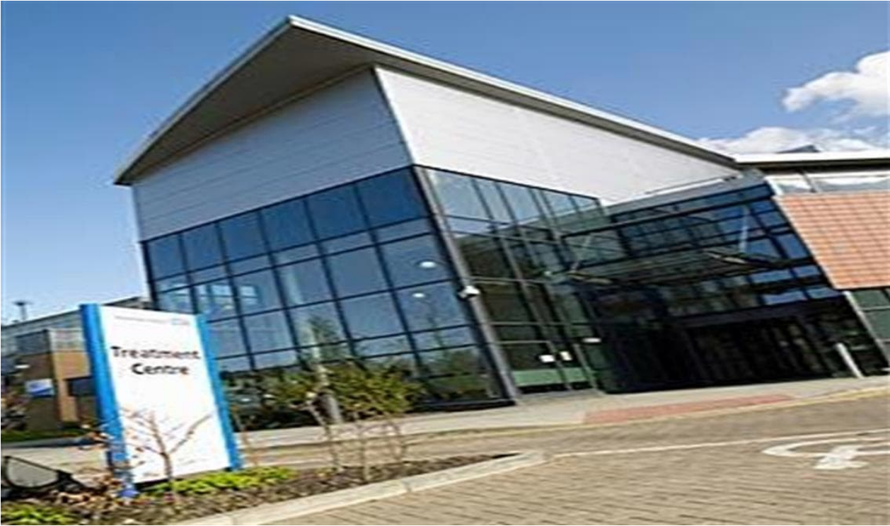
Ward Block 1, Good Hope Hospital - Sutton Coldfield, West Midlands
