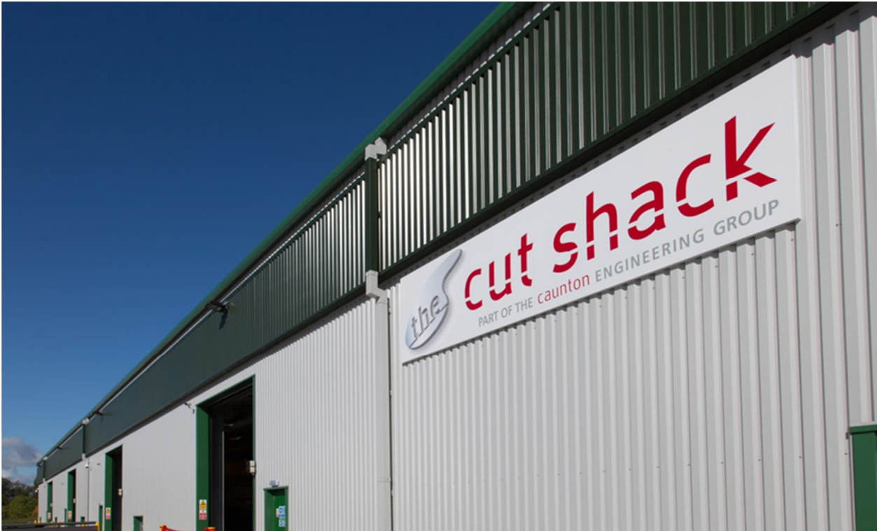
Project Hawthorn, The Cut Shack - Moorgreen, Nottingham
